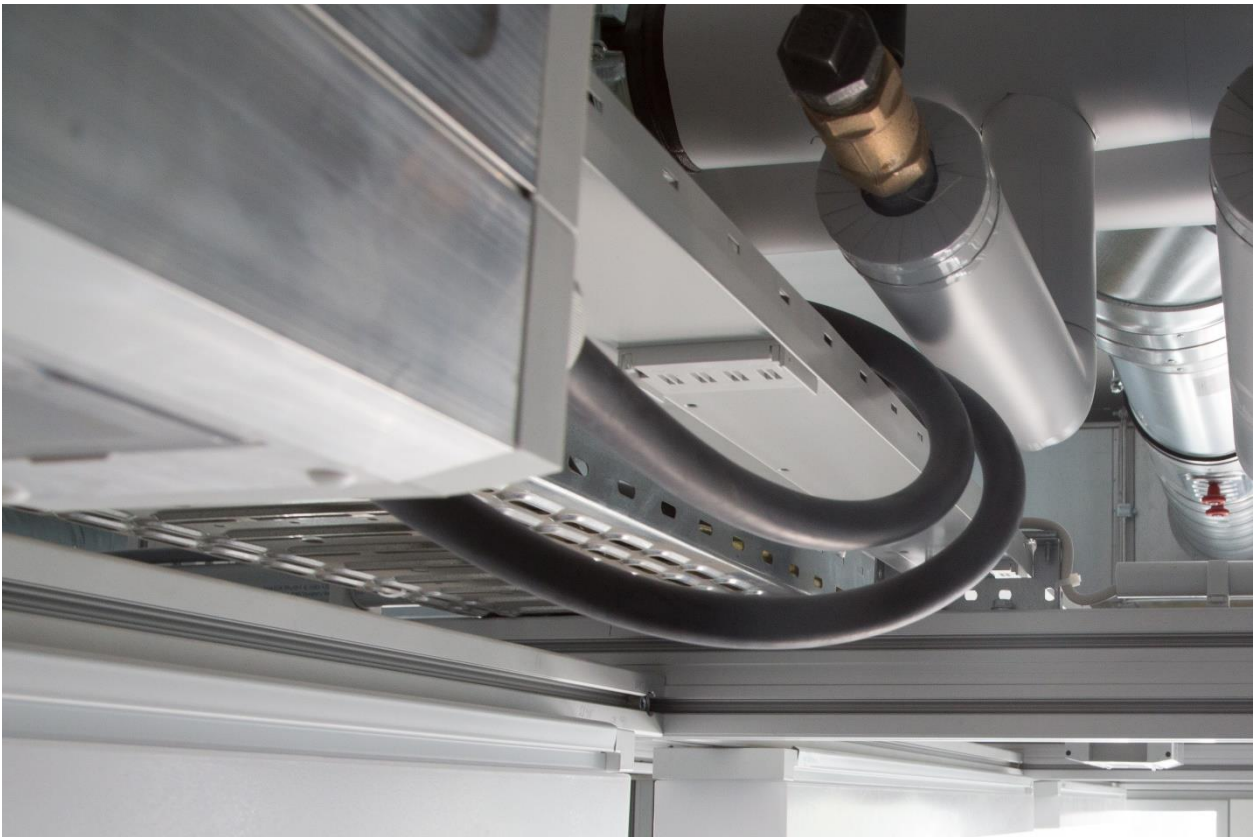
Bus bar with Connection Box for Media Column
